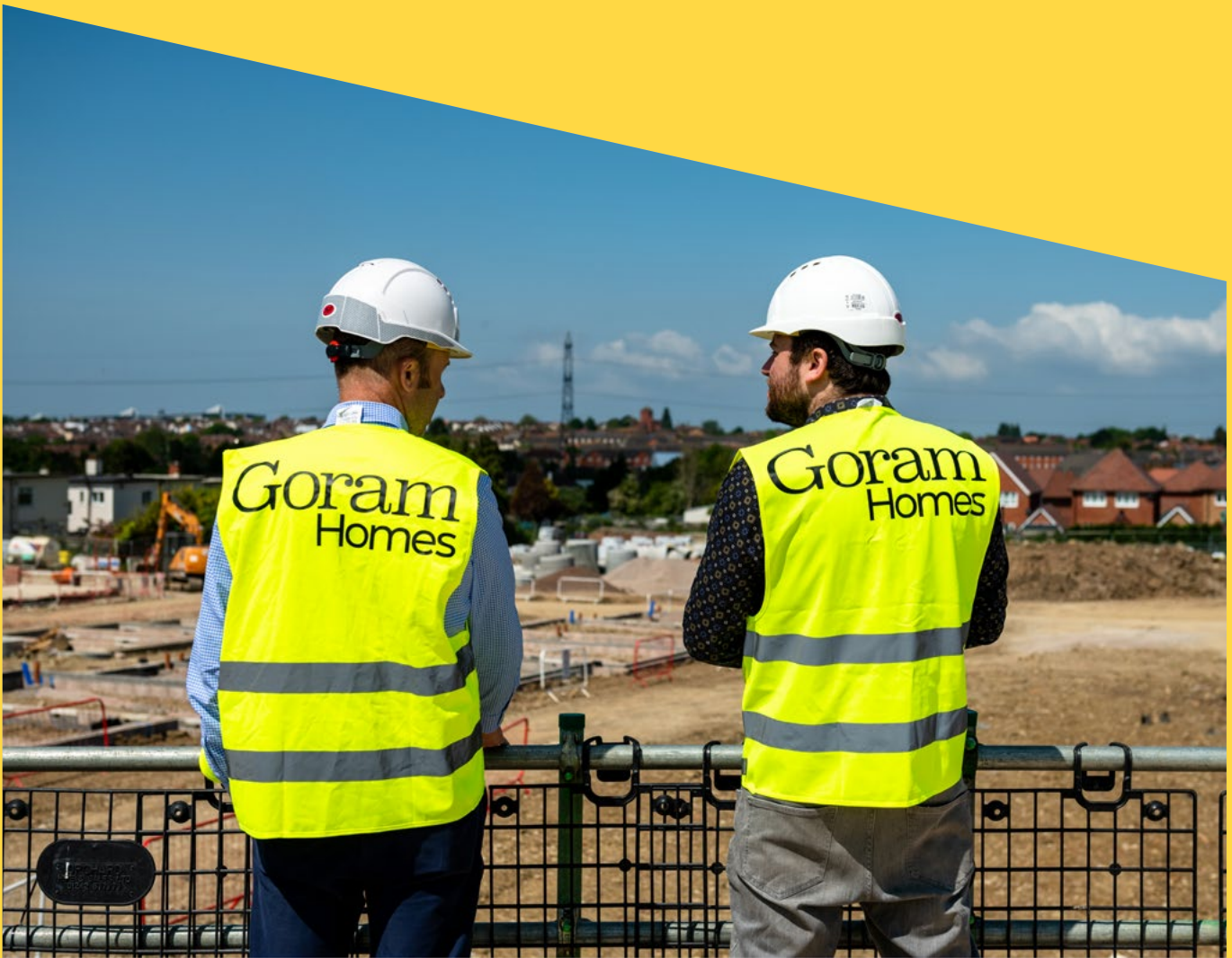
Credit: Rebecca Noakes Surveying progress at One Lockleaze in spring 2023.
