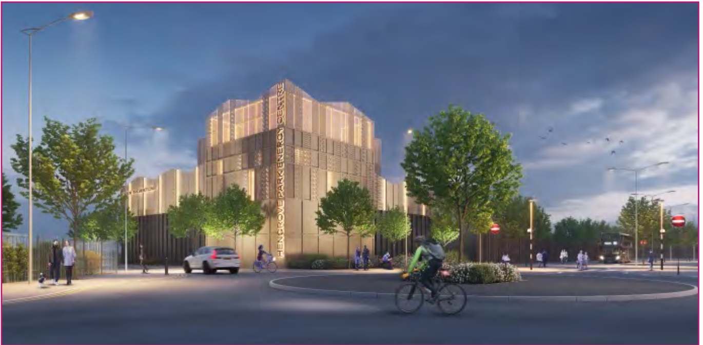
We're building an energy centre on our site at Hengrove Park
